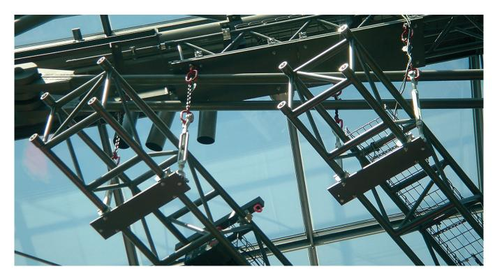
S36 Series truss is constructed of main chords (50 x 4 mm) and diagonal members (25 x 3 mm), and uses the CCS7 coupling system. Prolyte supplies a variety of S36 truss elements that provide maximum flexibility, including standard or custom-made lengths, circles and arches and several types of corners.
